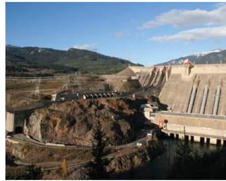
The Mica Dam near Revelstoke has a generating capacity of 1,700 MW; it is operated by BC Hydro.
