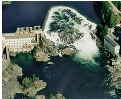
Nelson Hydro generating station (right) operating since 1907 at Bonnington Falls; Fortis BC plant (left). Source: Nelson Hydro, City of Nelson
