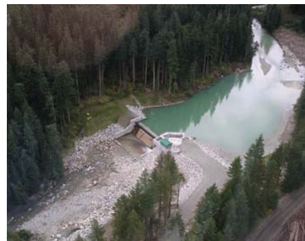
Aerial view of the head pond and weir at the Rutherford Creek run-of-river project near Pemberton.
